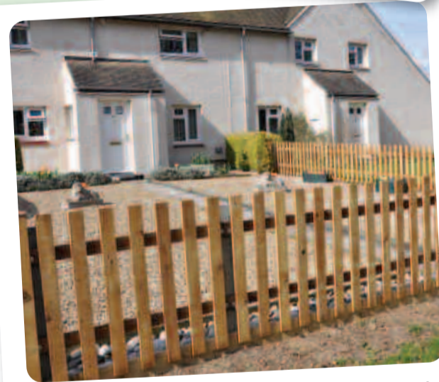
200 homes have had new fencing and 145 homes now have upgraded heating
