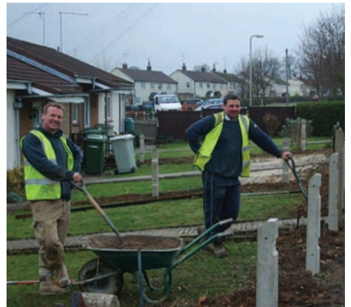
Contractors erecting new fencing
